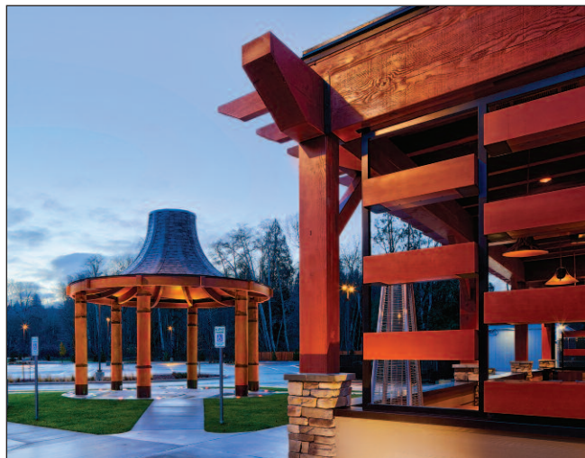
Traditional salmon bake structure
