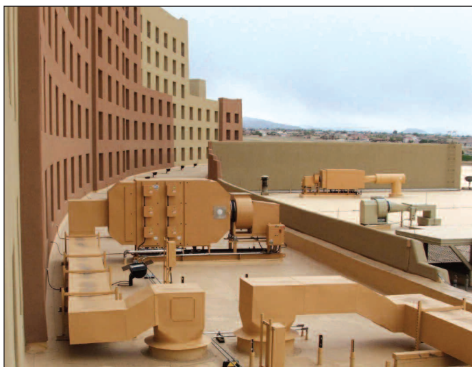
Shown on the roof at Sandia Resort and Casino, the Smog-Hog is a two-stage electrostatic precipitator.
